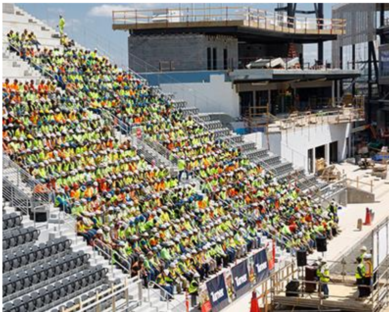
Construction workers stand-down to learn about fall prevention at a May 7 kick-off event held in the new DC United soccer stadium.
