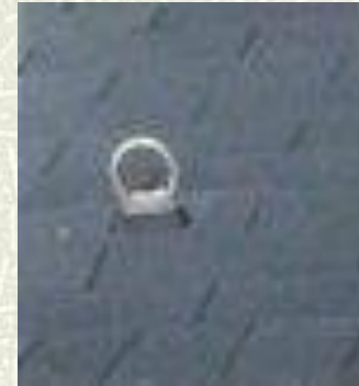
Wood Roof Anchor
